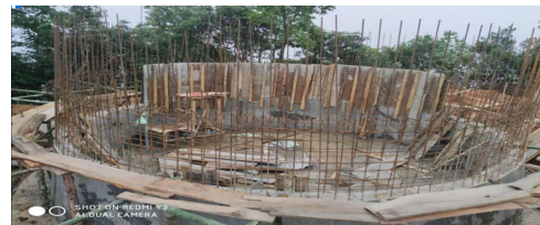
Figure 5. Deep boring under construction
