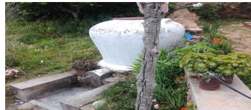
Figure 4. Rainwater harvesting tank
