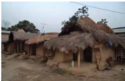
Traditional single-storey houses constructed facing north and south
