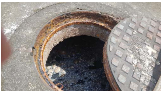
Fig. 6 Anaerobic reactor as seen through manhole
