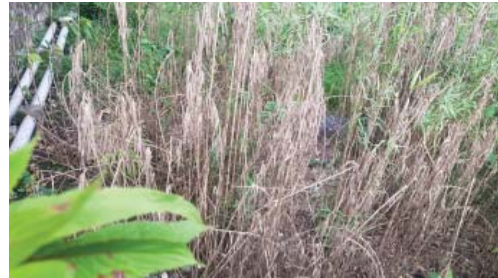
Fig. 7 HFCW -1 (Dry inlet pipe, withered reed plant and deposition of sludge)
