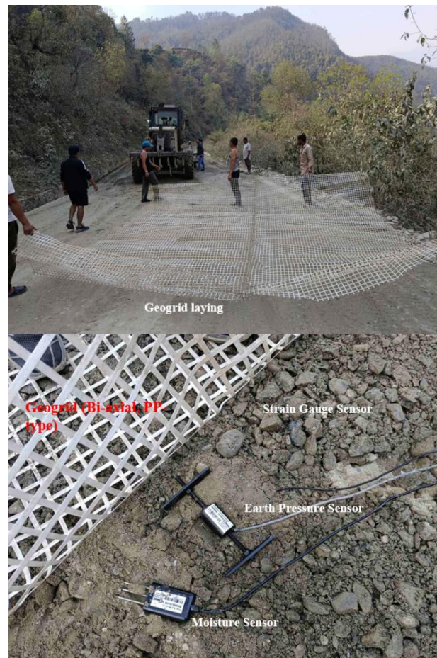
Fig. 3. Placement of Geogrid and Sensors: Left Fig.-40/40Q Biaxial Polypropylene Geogrid (Tensar); Right Fig.-Sensors beneath Geogrid at Mid-Depth of Base Course
