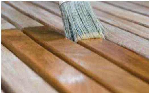
Plate 5: Preservation of Timber (Anupoju, 2021) Foundation Installation
