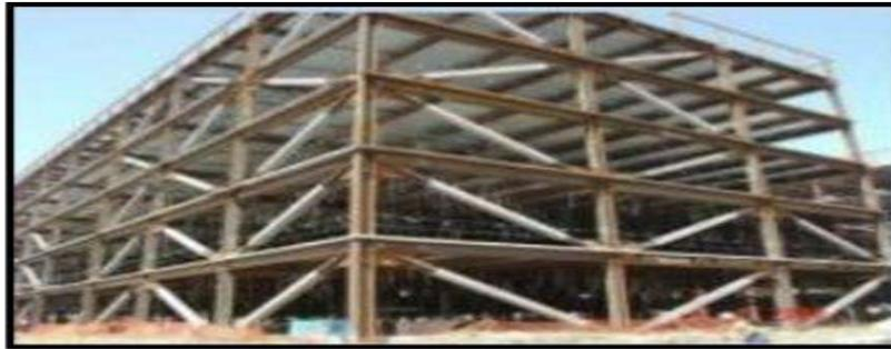
Figure 1.3: Seismic retrofitting by expansion of bracings
