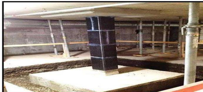
Figure 1.8: Retrofitting by Composite Fiber Wrap
