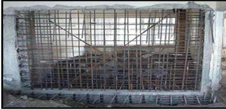
Figure 1.2: Seismic retrofitting by expansion of shear divider
