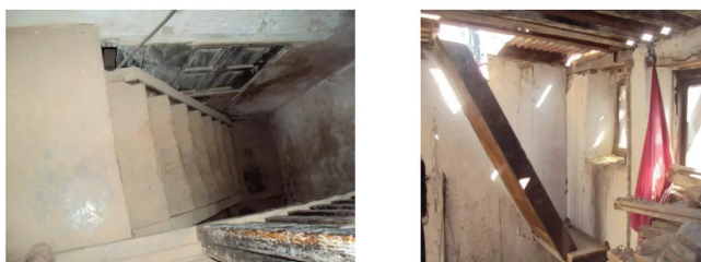
Fig XX: Staircase of First and Second Floor
