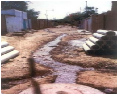
Figure 4. Internal sewer lane before, source: Hasan, 2011
