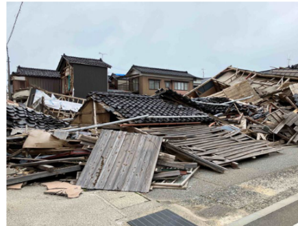
Figure 4: Collapse of traditional wooden houses in the epicentral area (Waima City)
