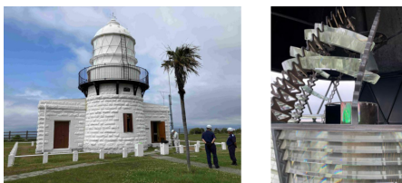
Figure 12: Rokko Cape Light house and its damage of equipment
