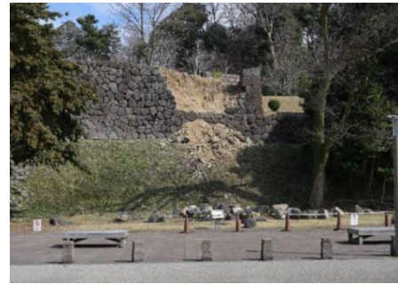
Figure 14: Collapse of stone retaining wall in Kanazawa Castle
