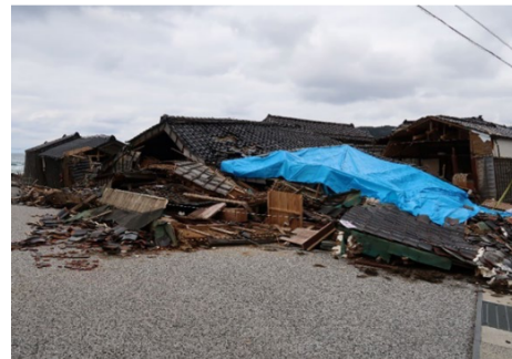
(b) After Earthquake
