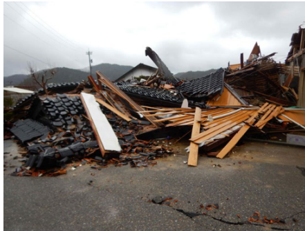
Figure 4: Collapse of traditional wooden houses in the epicentral area (Waima City)
