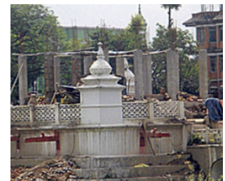
(b) Erection of cement pillar
