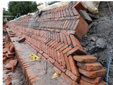
Figure 6: Construction of embankment wall
