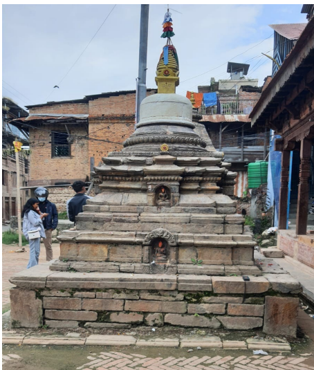
Figure 6. Chaitya after relocation
