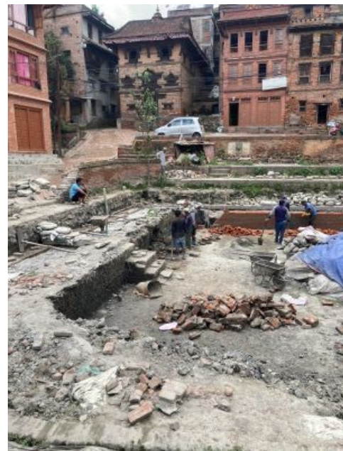
Figure 12. Restoration work of Salanpukhu (Bhaktapur)
