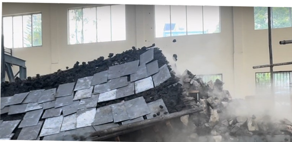
Figure 17. Roof impact splits the roof along the ridge beam and causes slate roofing to fly off.
