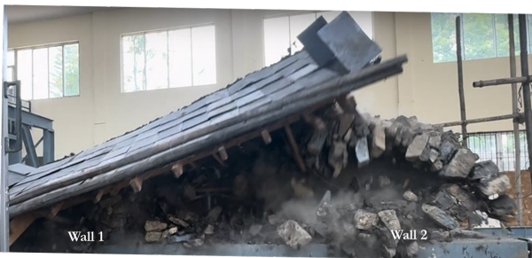
Figure 16. Collapse of wall 2 continues.
