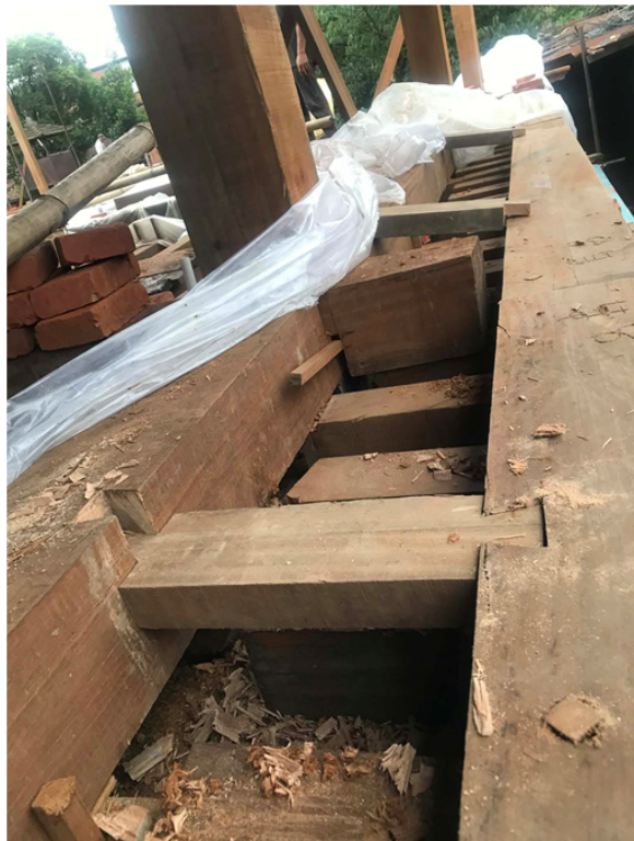
Figure 22. Horizontal sill and lintel band tie up
