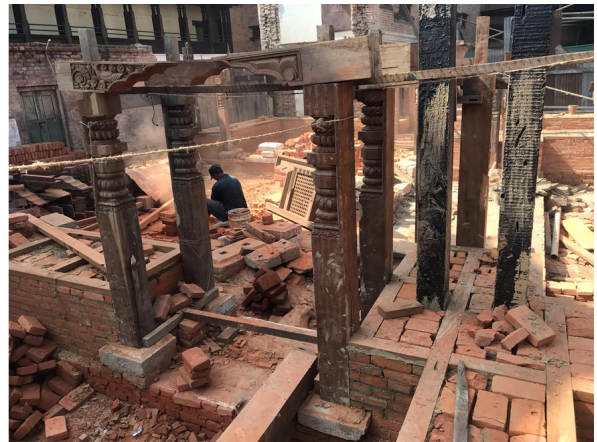
Figure 19. layout of post on base stone
