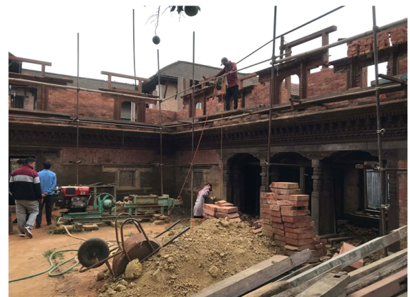
Figure 25. Ongoing reconstruction upto first level
