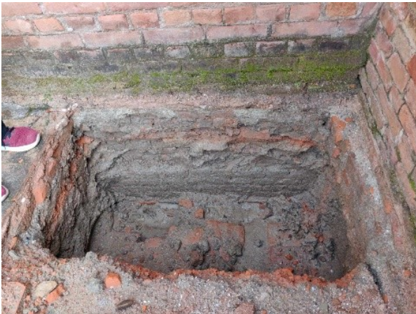
Figure 12. Pit excavation for foundation study 01
