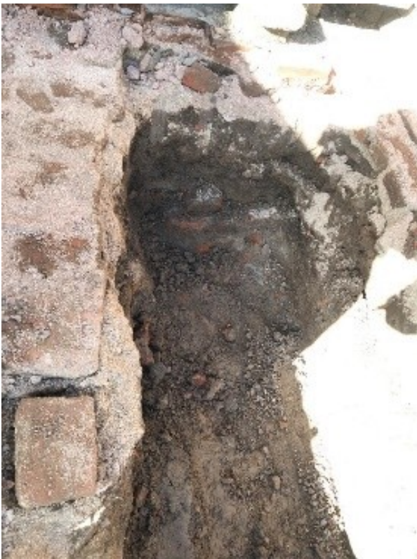
Figure 13. Pit excavation for foundation study 02
