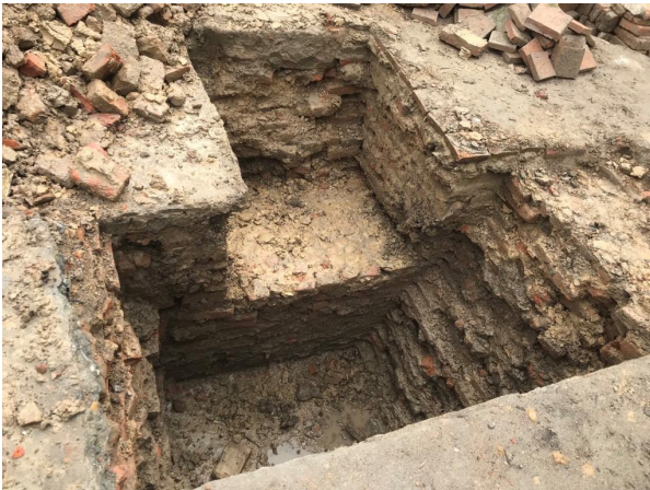
Figure 16. Pit excavation for foundation study 05
