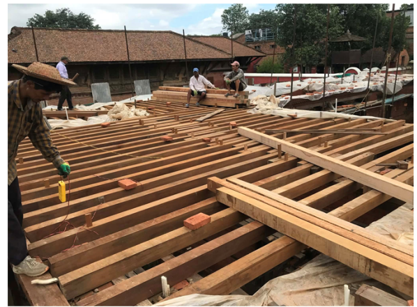
Figure 24. Wooden joists laying in first floor
