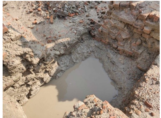
Figure 14. Pit excavation for foundation study 03
