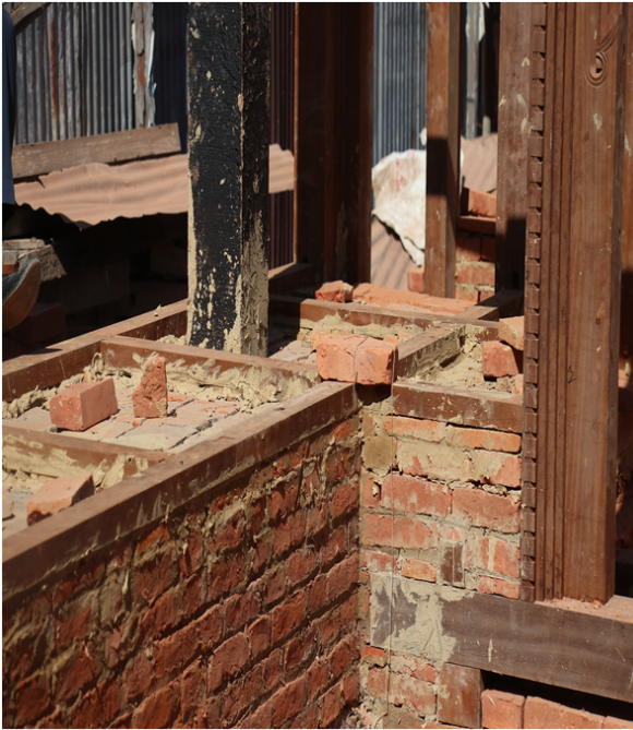
Figure 21. Horizontal sill and lintel band installation
