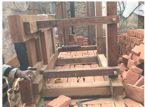
Figure 20. Opening installation with wooden joineries
