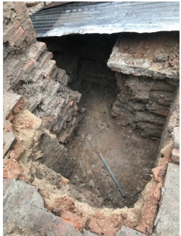
Figure 15. Pit excavation for foundation study 04
