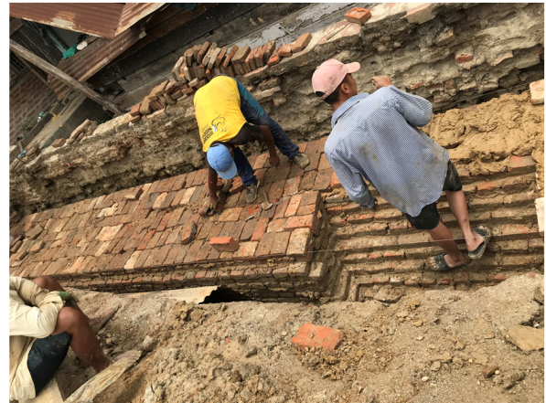
Figure 18. Foundation brick works
