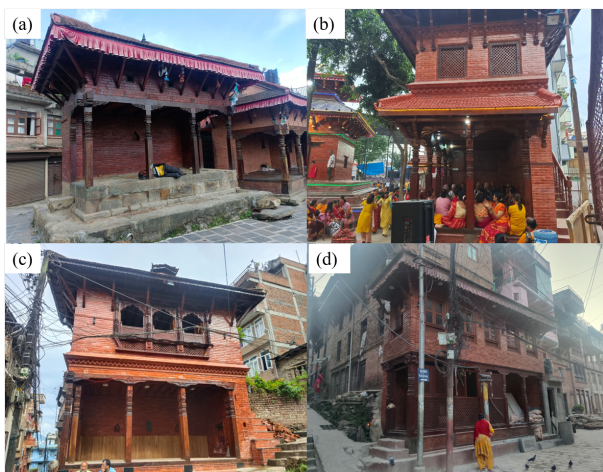
Figure 1. Typical resthouse (sattal/falcha) in Kirtipur showing different wall and frame layout positions at (a) Devdhoka (b) Sundarbasti (c) Kutusagal and (d) Kutujho
