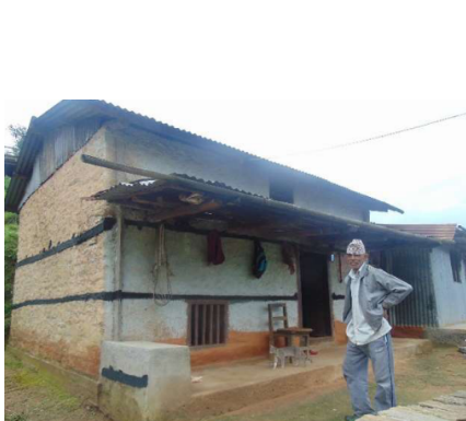
(c) Post-earthquake demo house replication (Source: ASF Nepal)
