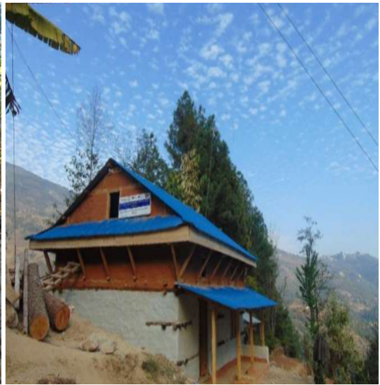
(b) Post-earthquake demo house (Photo: ASF Nepal)
