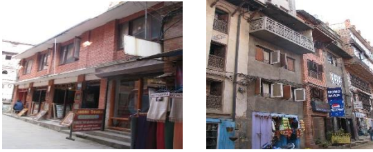
Fig. 9. Brick masonry with cement mortar (BC)
