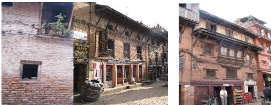
Fig. 10. Brick masonry buildings with mud joints (BM)
