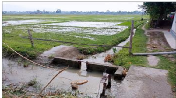
d) Damaged regulating structures
