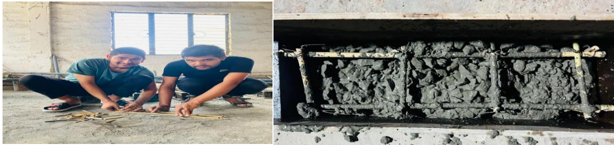
Figure 4: Nigalo reinforcement preparation and casting of NRC Beam
