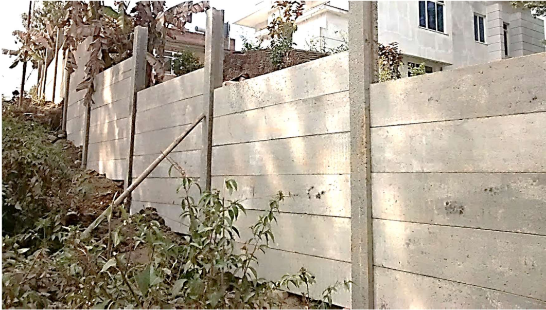
Figure 1: Boundary wall constructed with H-post and panels
