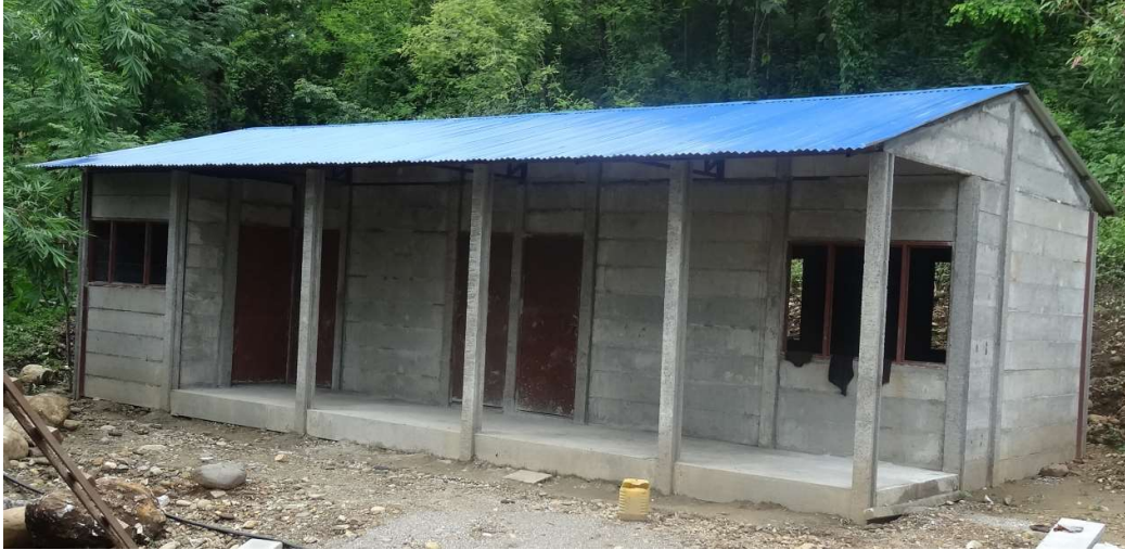
Figure 2: A shed constructed using H-post and panels
