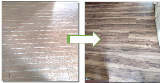
Figure 11: Flooring material changed from tiles to parquet
