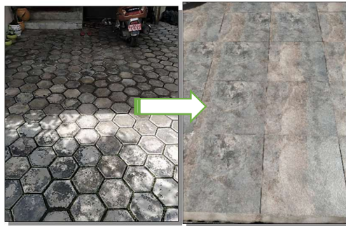
Figure 12: Concrete block parking tiles changes into vitrified parking tiles
