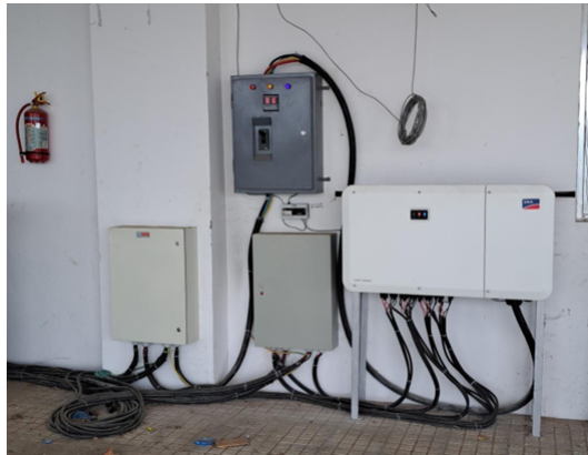
Figure 2: SUNNY TRIPOWER STP CORE 2 installed at site[6]
