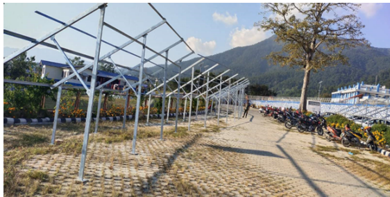
Figure: Part of PV array mounting structures of 150kWp On-grid solar PV system[5]
