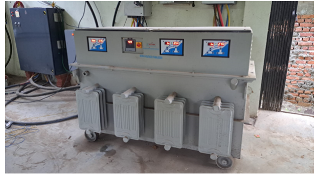
Figure: Voltage Stabilizer installed for PSA plant[6]
