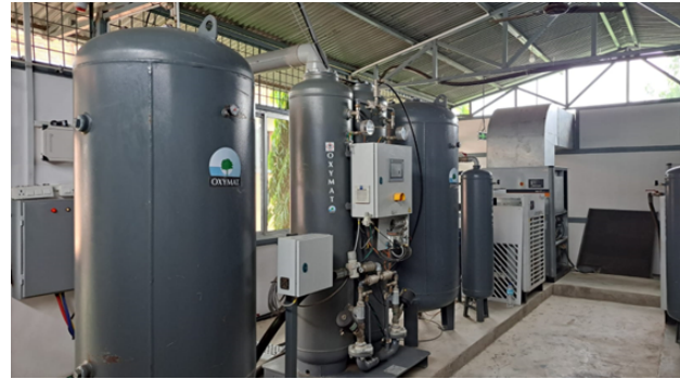
Figure: PSA plant installed at hospital
