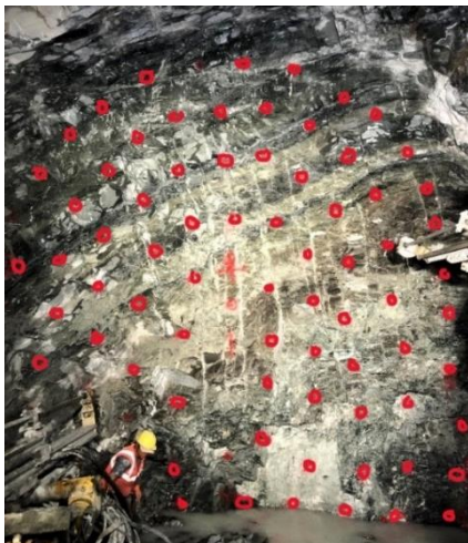
Figure 3: Marking for drilling
