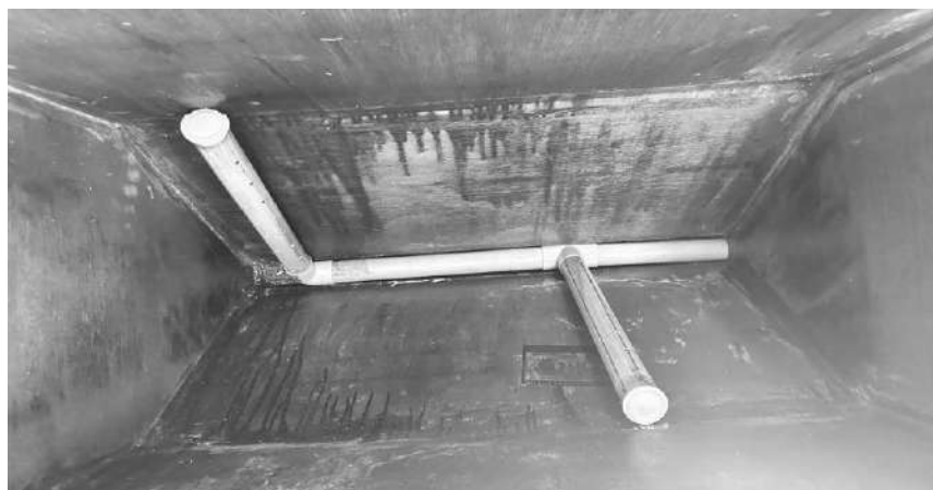
Figure 1. Perforated Pipes in Desilting Basin
