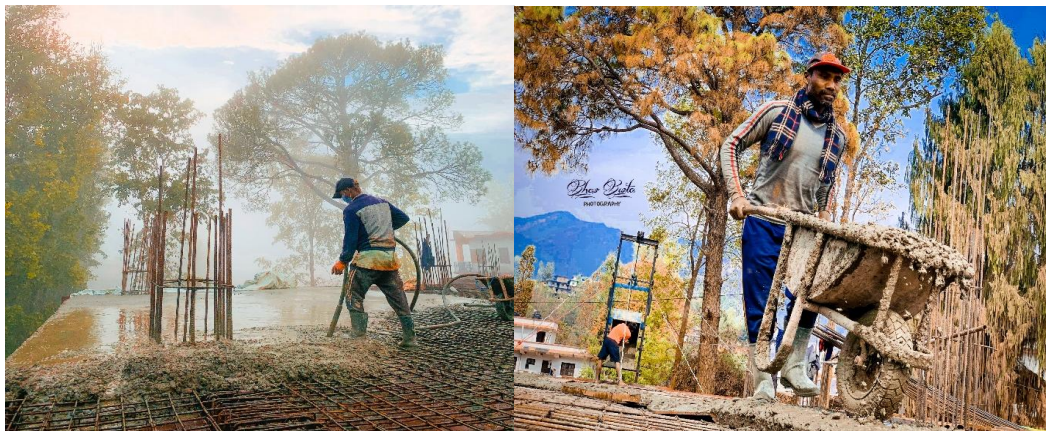
Figure 3: Construction workers working in both sunny and foggy weather
