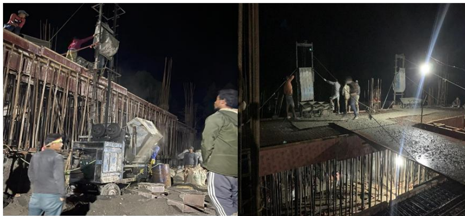
Figure 3: Late night work done by construction labours
