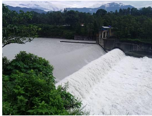
Figure 5: An image showing an example flow over the weir at Tulsighat
