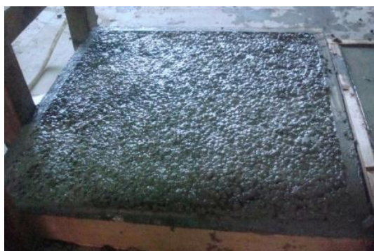
Figure 5: Casting Condition of EPS Panel
