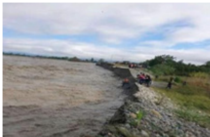
Mahakali River Sidecutting
