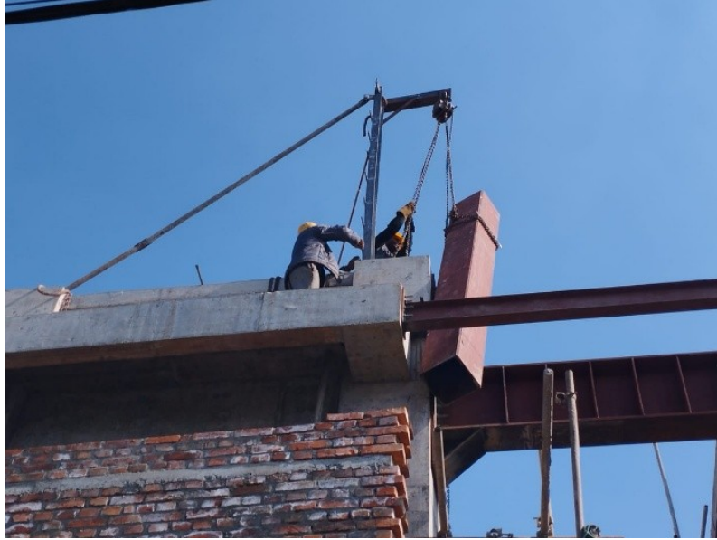
FIGURE 5. Erection of 2 ISMC column (toe to toe connection)
