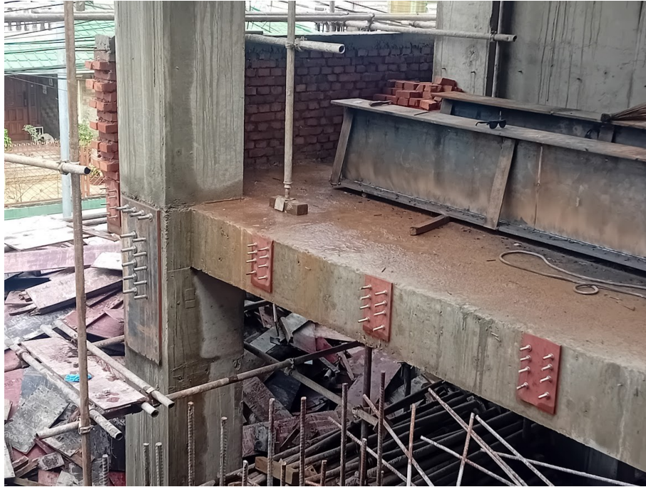
FIGURE 11. Installation of base plate prior to PEB beam installation
