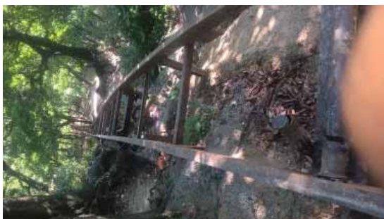
Fig 7. shows a rail structure which was used to carry construction materials in one of the temples of Pashupati jungle.
