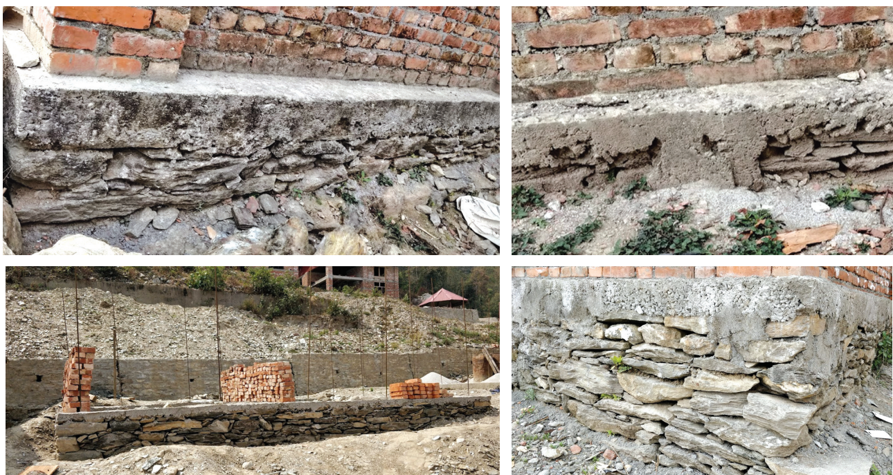
Figure 14. The plinth wall construction in dry stone
