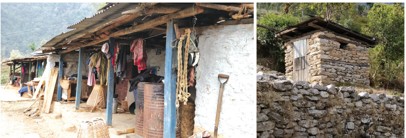
Figure 3. (a) Ground floor of old building was retained for continued use (b) Reconstructed toilet block with some timber reinforcement.
