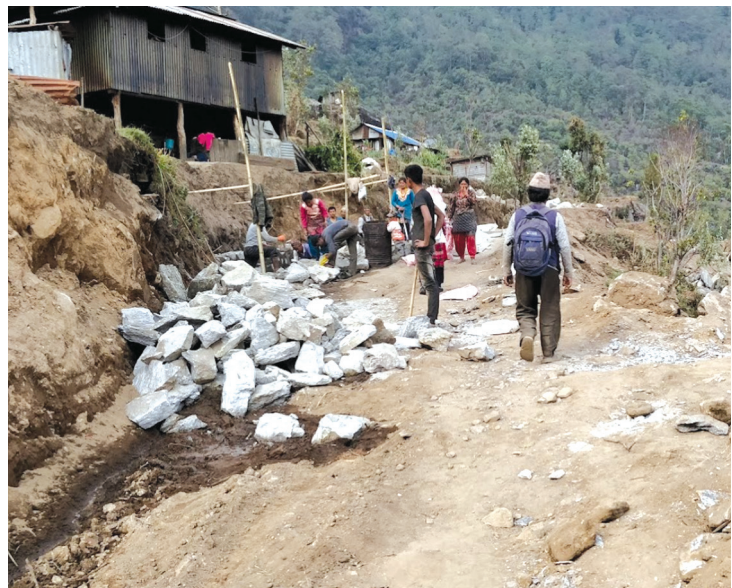
Figure 6. Ongoing road construction in old settlement.
