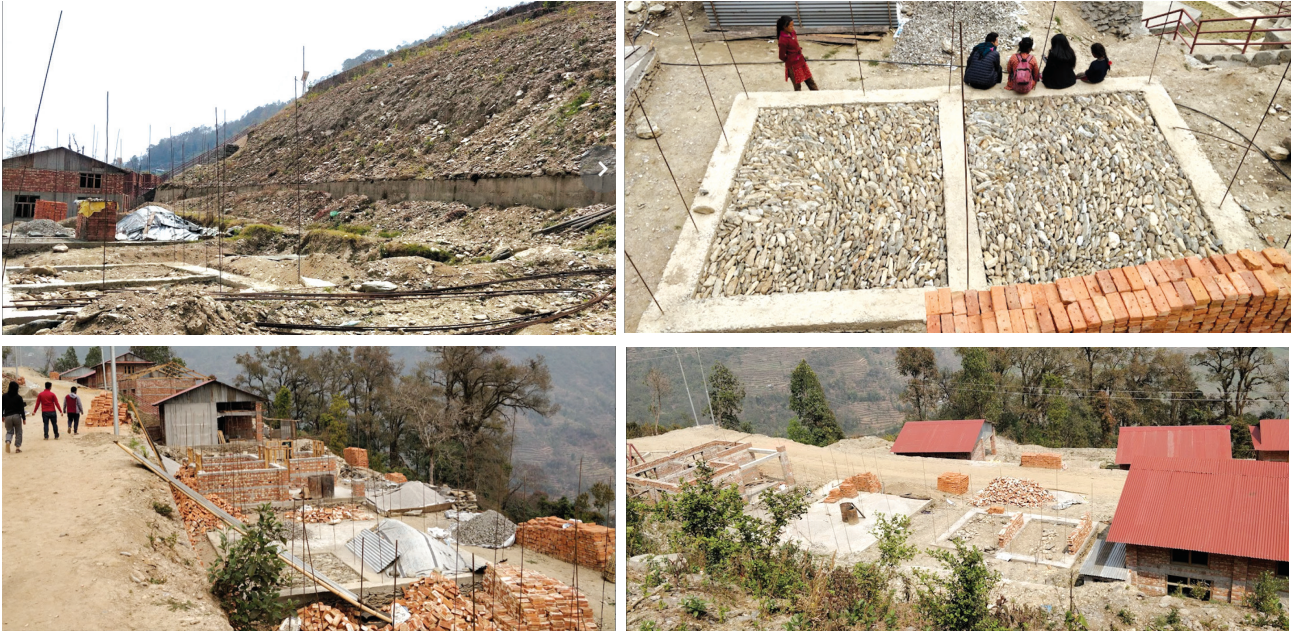
Figure 15. Plinth beam construction and laying of vertical rebars
