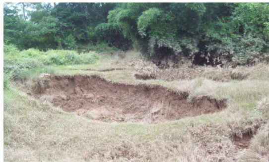
Photo 1: Sinkhole formation on Davis Fall Area (Photo by Author taken on Aug.18, 2014)
