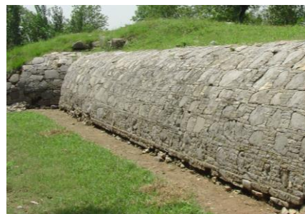
b. Original Boundary wall at Taxila
