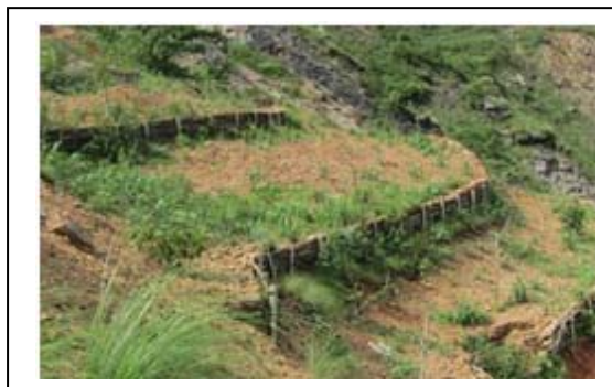
Fig. 6: Landslide mitigation measure at the source area.
