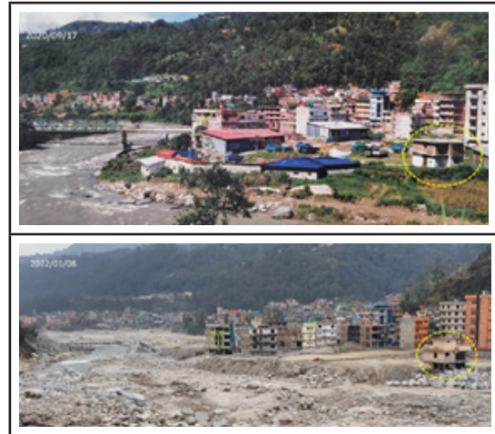
Figure 2: Melamchi bazar before and after flood: (Source: WB & GFDRR, 2022)
