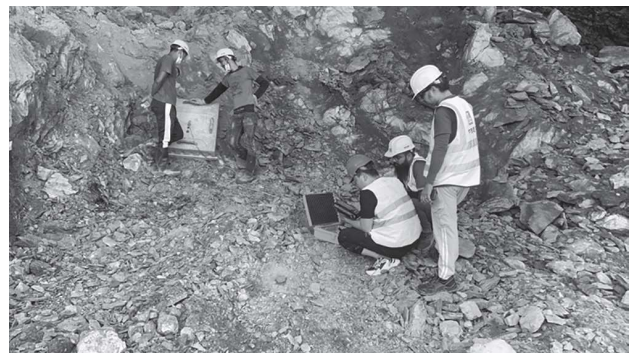
Figure 3: Conducting GPR survey in Mahadevtar tunnel
