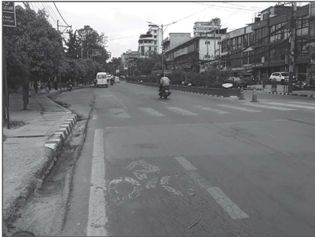
Figure 9: Erased road marks of zebra crossing and cycle lane at Pulchowk, Lalitpur
