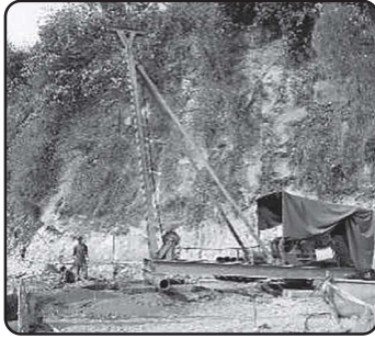
Figure 8: Impact Boring
