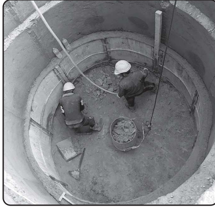
Figure 2: Mucking in manual hole excavation
