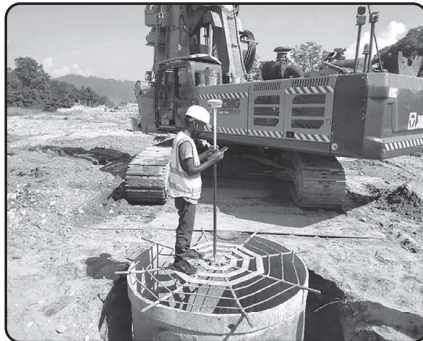
Figure 6: Survey and Setting Out
