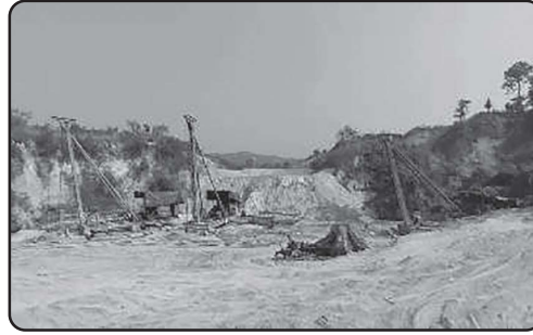
Figure 9: Several Percussion machine for boring
