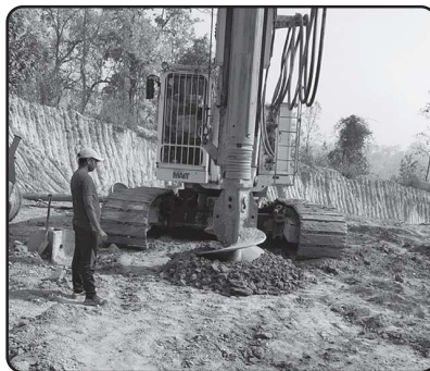
Figure 5: drilling machine in place
