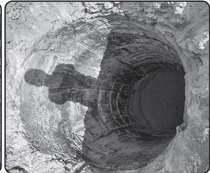
Figure 7: Dry hole boring
