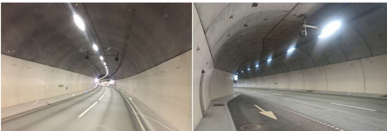
Fig. 9: Water shielding. Left: combination of shotcrete and polyurethan foam (PE-foam) on the roof and concrete elements in the walls and right: combination of concrete elements and waterproofing membrane.
