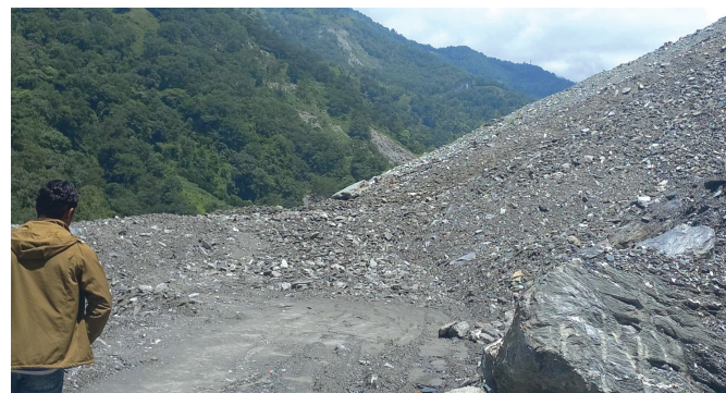
Fig. 3: The debris of Bukula landslide disturbing access road of hydropower project.
