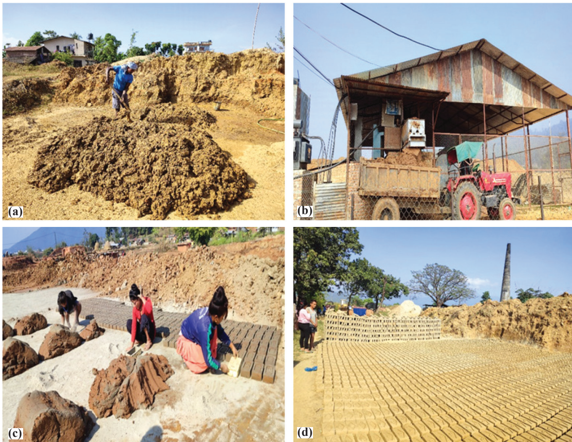
Fig. 3: Field observation of brick manufacturing sites; (a) manual pugging, (b) mechanized pugging, (c) moulding, (d) drying and stacking.
