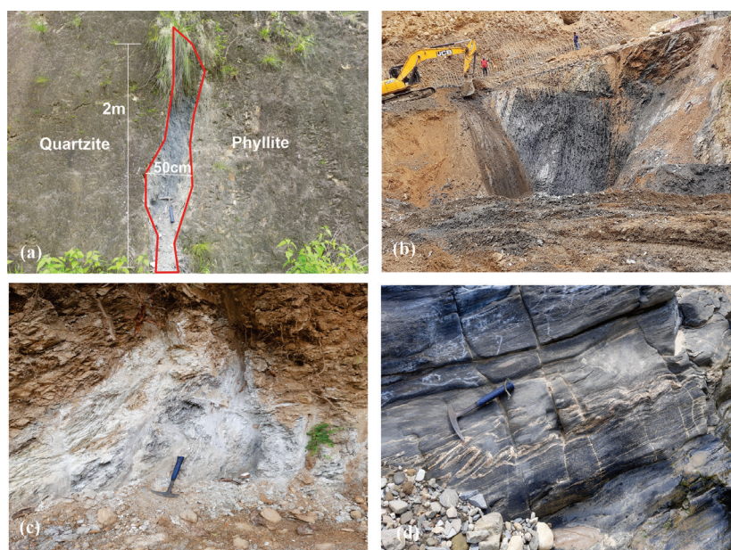
Fig. 9: Crushed zones (a) observed in the Benighat Slate along the Arniko Highway near Dhondra Khola (view towards west), (b) observed in the Benighat Slate at Maitar (view towards west), (c) crushed zone observed in the Benighat Slate along Sipaghat-Sakhu Road section (view towards south), (d) boudinage structure observed in the Benighat Slate near Cha Khola (view towards north).
