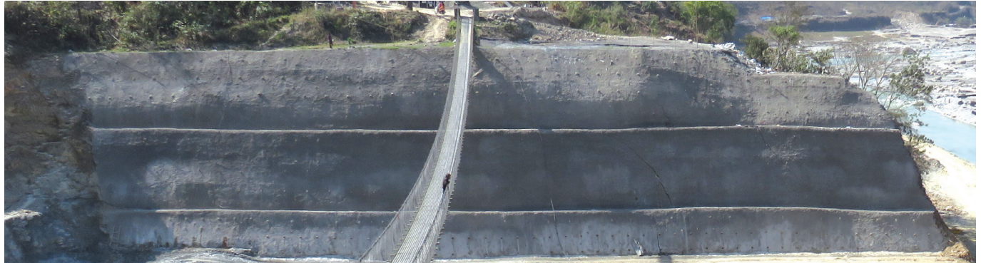
Fig. 2: Cut slope face of the desander basin in project area.
