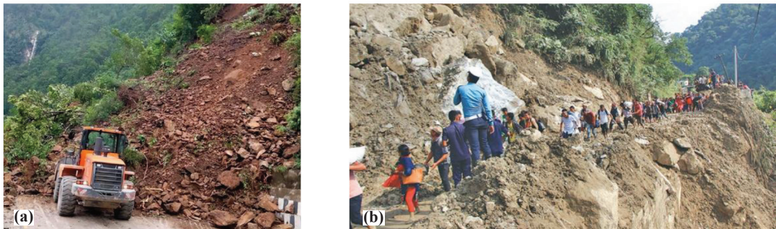
Fig. 2: Difficulties faced on roads of Nepal (a) landslide on Pokhara Baglung Highway (Nepal Press, 2021), (b) landslide on Siddhartha Highway (Kathmandu Post, 2017).
