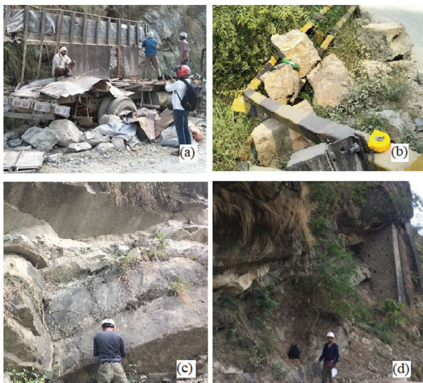
Fig. 7: Field photographs (a) A truck hit by rock-fall at zone 15, (b) Bending of beam due to rock-fall at zone 17, (c) Data collection during the field d) Measurement of length of different zones.
