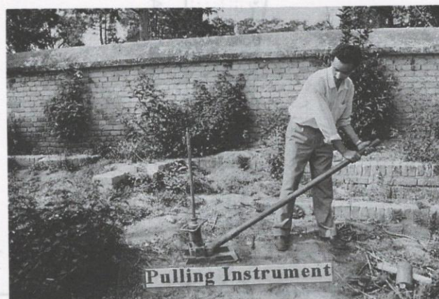
Plate 1b: Method of extracting the rod from the ground
