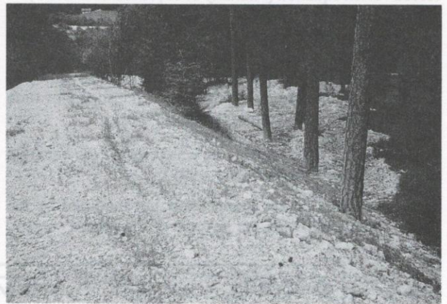
Plate 8: Debris overflow beyond the dyke. The torrent Fojedöra is to the left of the dyke.
