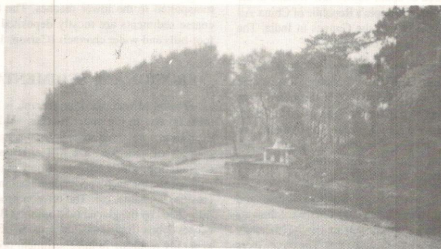
Fig. 1: Down stream view of Lothar river showing bio-engineering works on right embankment and series of short sloping spurs.
