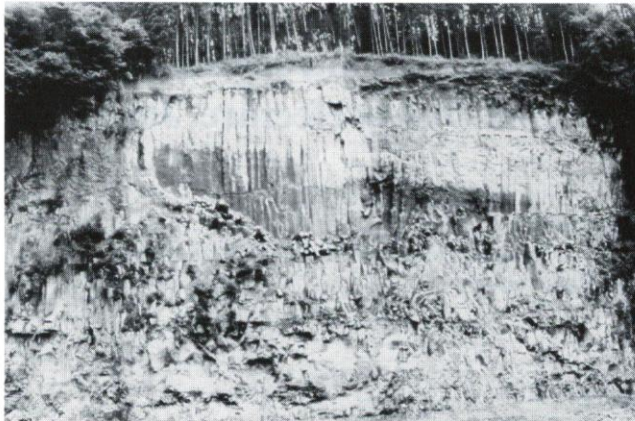
Fig. 1: Photograph showing the rock mass (welded tuff) of the slope.
