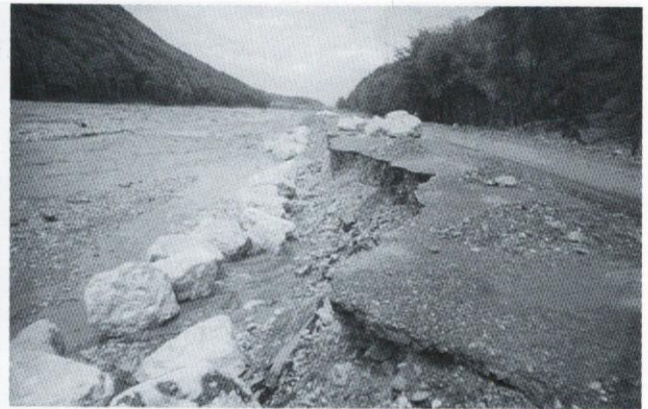
Fig. 7: Right bank of Gizeldon River down the Genaldon River mouth. Debacle of 16 June 2003 has destroyed the road. Photo by E. Zaporozhchenko
