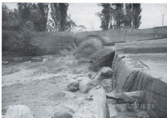
Fig. 9: Flood (with a discharge of about 30 \text{ m}^3/\text{sec} ) through Gizel Hydro-Engineering complex. Photo by E. Zaporozhchenko, 16 June 2003
